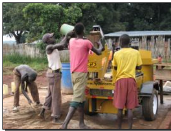
Making our own blocks for the buildings at Bori.
