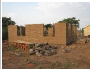
Guest house for farmers under construction at Bori.
