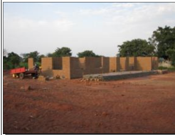
Bori Mill under construction.
