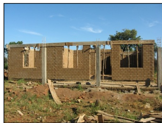
Volunteer guest house at Bori ready for the roof.
