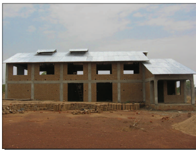
Mill House ready for equipment
