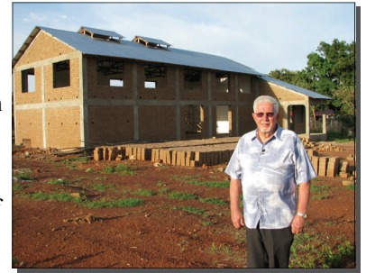
The mill building is ready for the installation of the equipment
