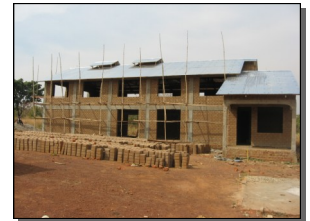
Bori mill under construction
