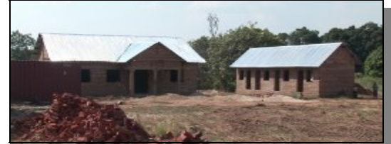
New Central Compound offices and guest house Under construction
