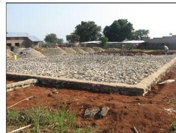
Church foundation being laid
