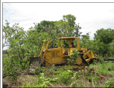
Land clearing in heavy brush
