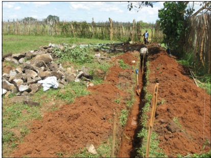
Foundation for compound wall
