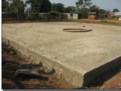
Workshop floor is completed
